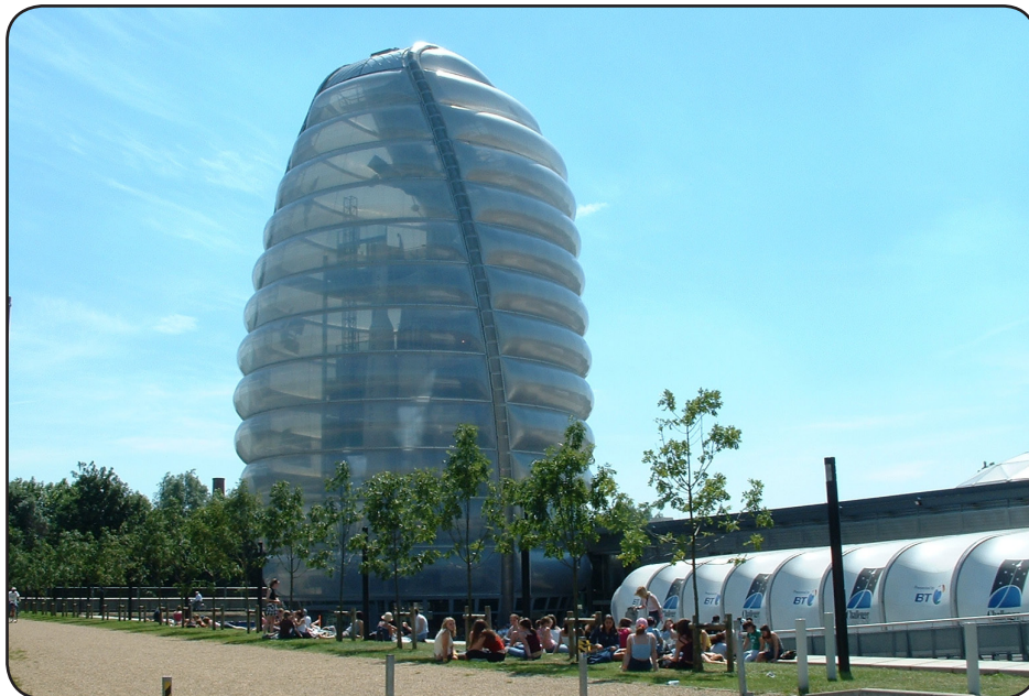
Figure 13 National Space Centre.
